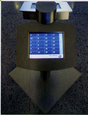
Destination-based dispatch software can reduce energy use by coordinating elevator rides
